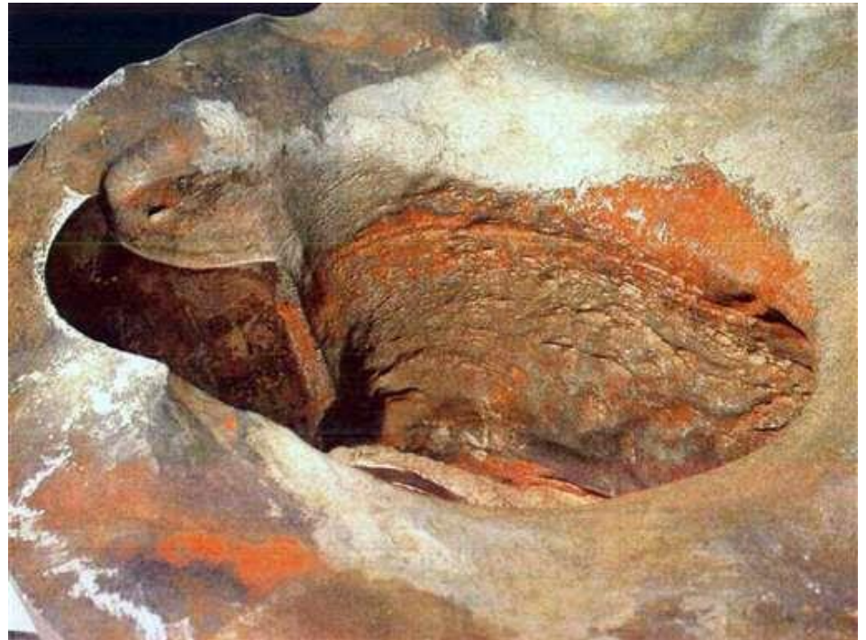
Davis-Besse reactor vessel head degradation
